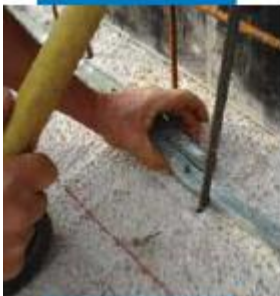
Fixing Idrostop B25 in place
